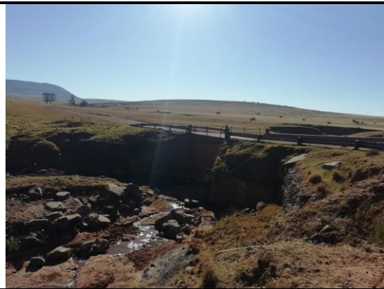
North western view of the bridge over the Mjanyana River.
