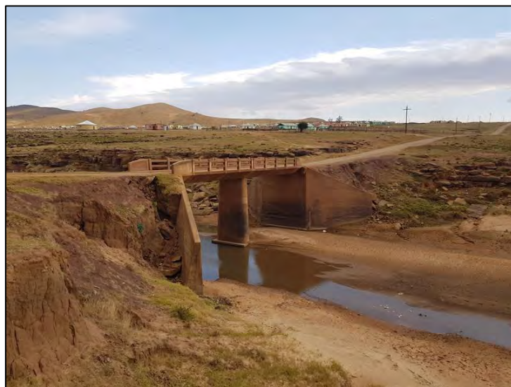
Figure 3-8: View of an existing road culvert in the Mtshayelweni area.
