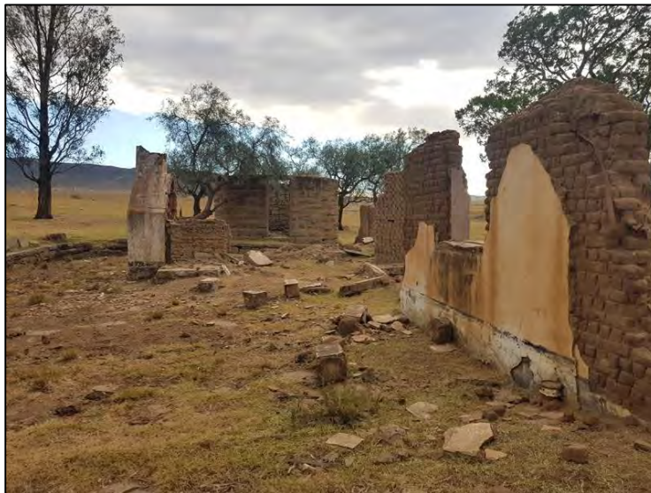
Figure 5-20: View of building remains remains at Site EXIGO-MCRU-HP04. Note the stone rondel in the middle background.
