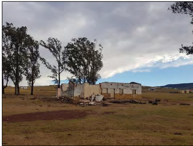
Figure 5-21: View of the remains of the Phillipsdale Trading Store at Site EXIGO-MCRU-HP04.
