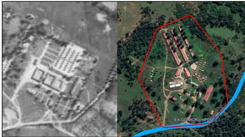
Figure 5-23: Site EXIGO-MCRU-HP05 (Mjanyana Leper Asylum and hospital) indicated on an archive aerial image (1938, left) and current aerial imagery (right).
