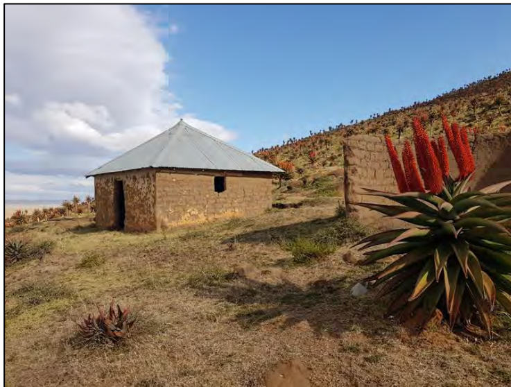
Figure 5-14: View of a mud brick dwelling and hut remains (right) at Site EXIGO-MCRU-HP03.
