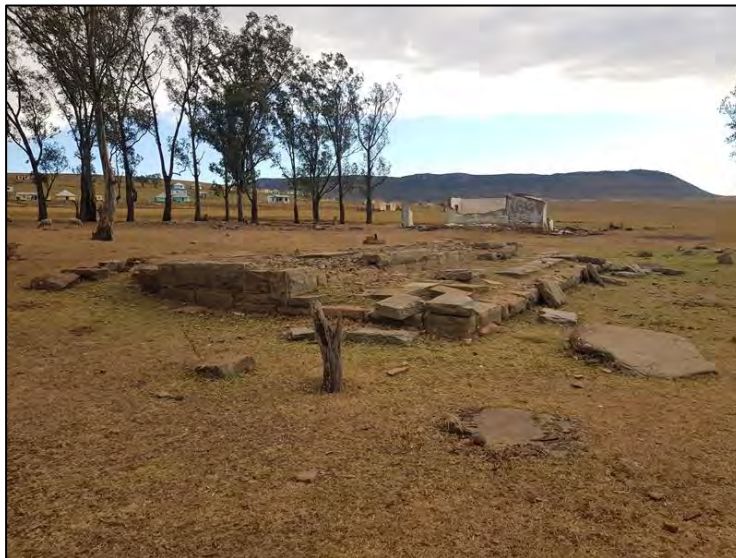
Figure 5-19: View of a sandstone building foundation at Site EXIGO-MCRU-HP04.
