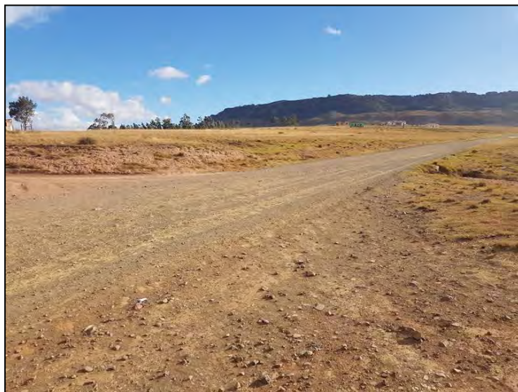
Figure 3-17: View of the western offset of the road upgrade alignment at Lookout.
