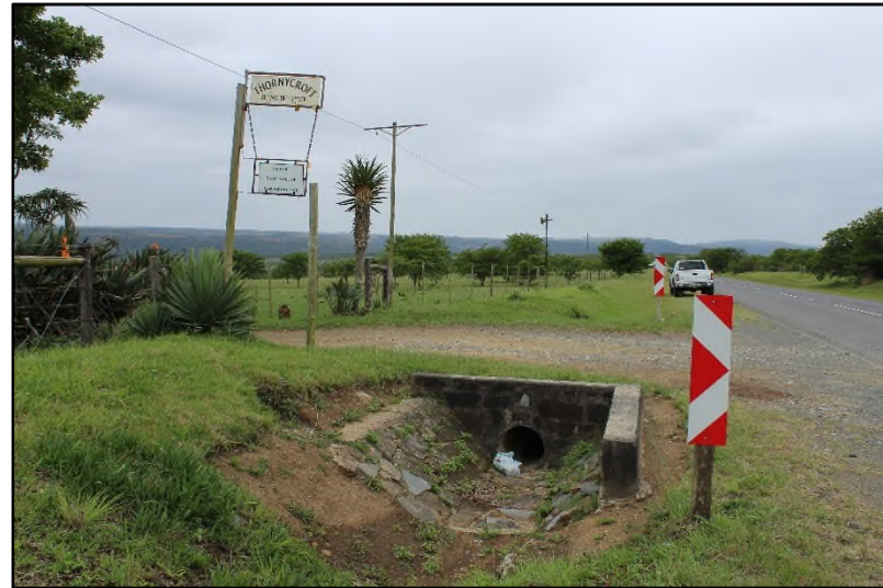
Plate 36: Stone paved culverts [1]
