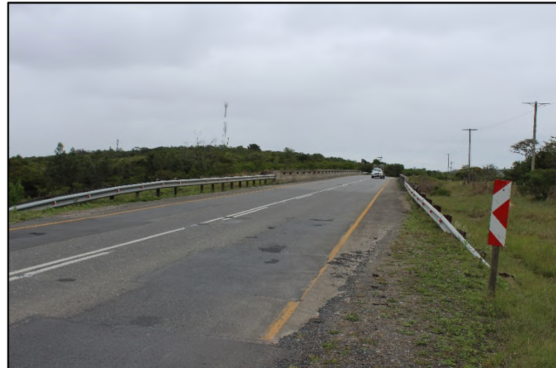
Plate 32: Selected bridges along the line route [1]
