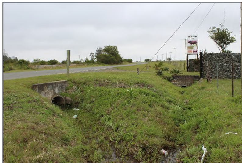
Plate 40: Stone paved culverts [5]
