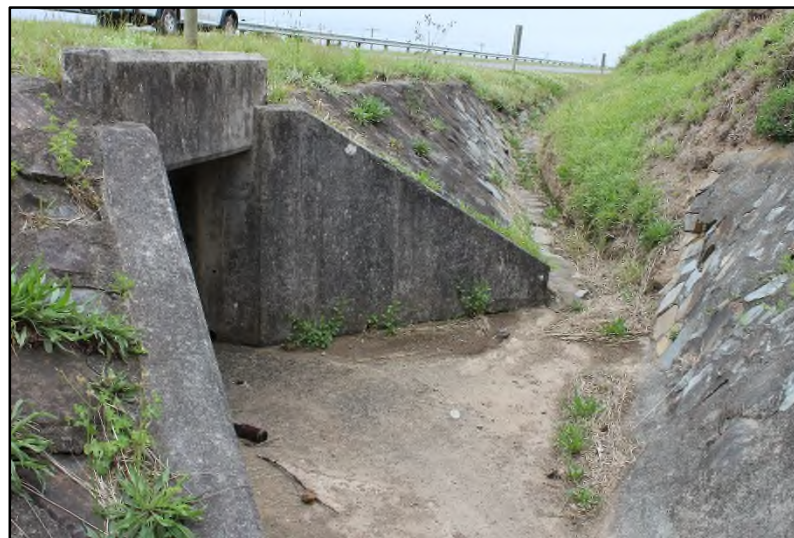
Plate 39: Stone paved culverts [4]
