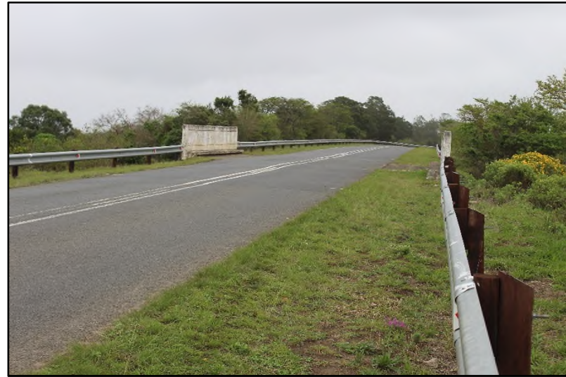
Plate 35: Selected bridges along the line route (rail bridge 2)
