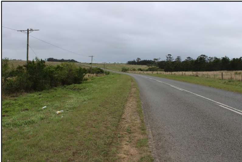
Plate 10: General view of the R63, Section 16, line route [2]
