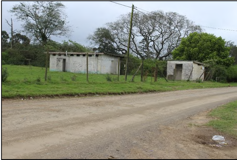
Plate 17: View of Site R63-S5
