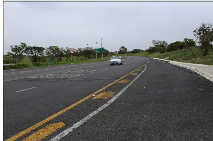
Plate 12: End of the R63, Section 16, line route at km 43,64
