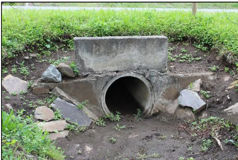
Plate 38: Stone paved culverts [3]
