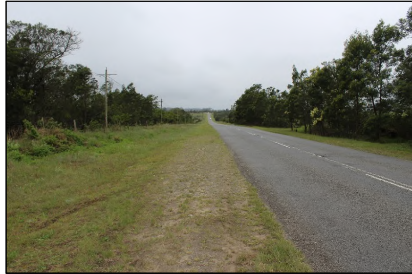
Plate 11: General view of the R63, Section 16, line route [3]
