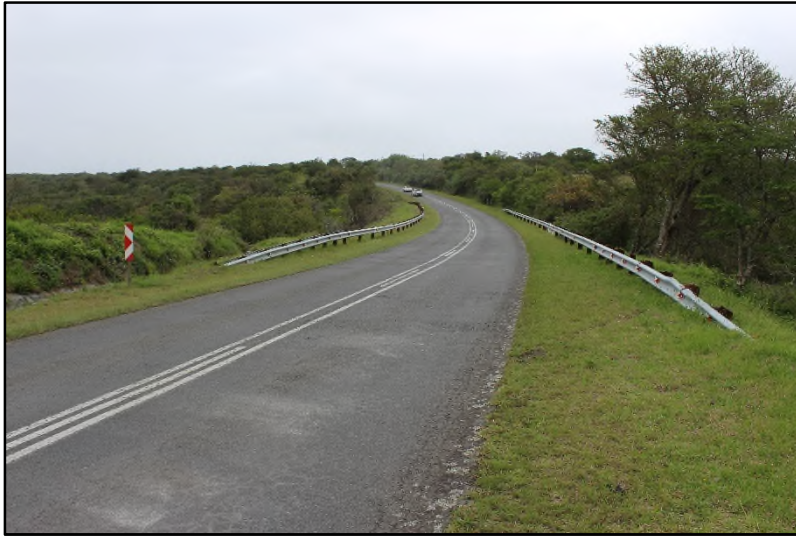
Plate 9: General view of the R63, Section 16, line route [1]
