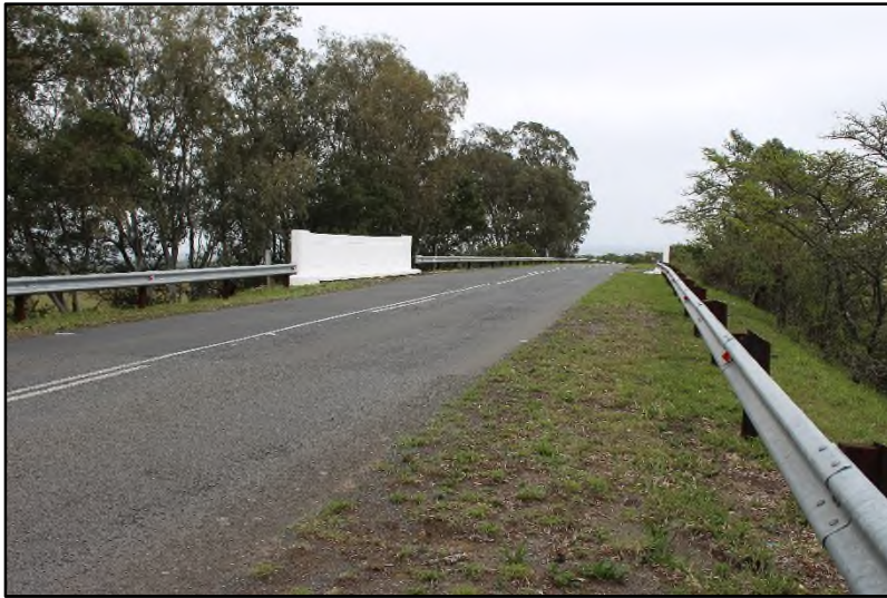
Plate 33: Selected bridges along the line route (rail bridge 1)
