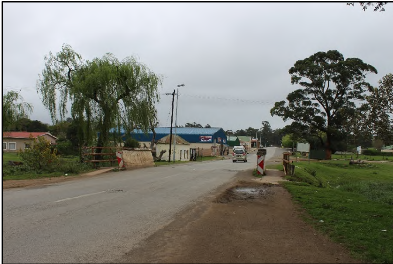
Plate 34: Selected bridges along the line route (bridge in Komga)
