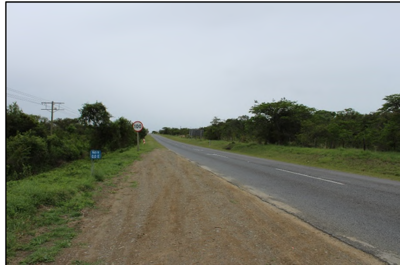
Plate 8: Start of the R63, Section 16, line route at km 1,00
