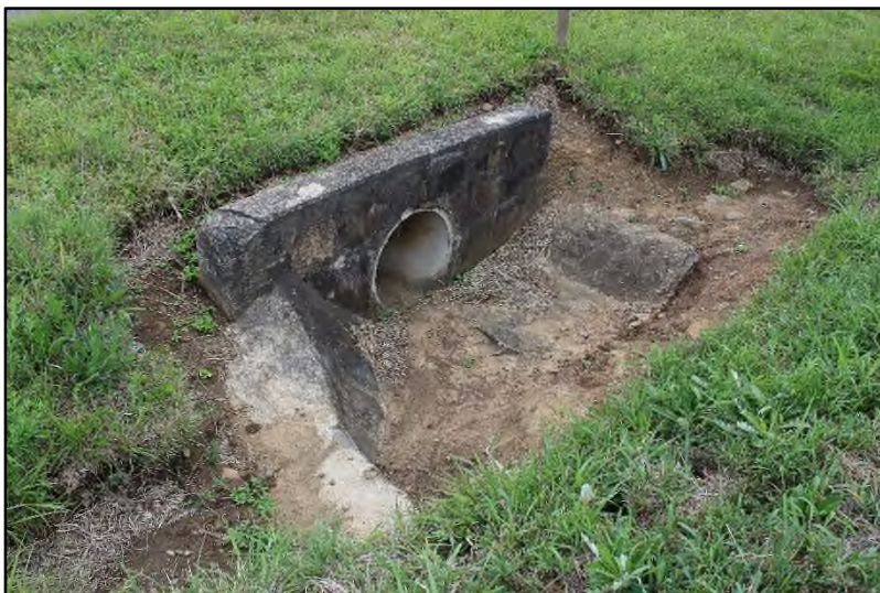
Plate 37: Stone paved culverts [2]
