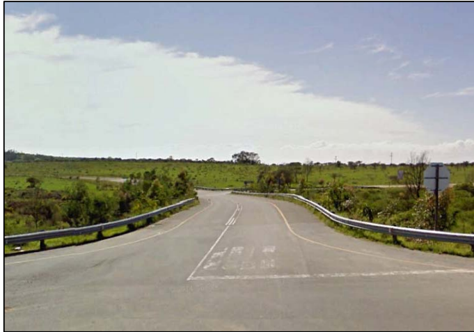
Photo 5: Eastbound view along MR694 from the R349
