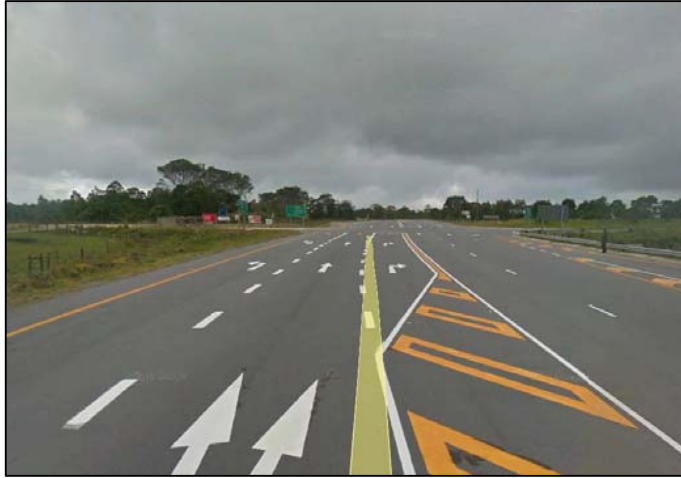
Photo 1: Northbound view along the N2 towards the R349 intersection
