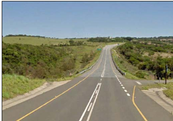
Photo 3: North westbound view along MR697 towards MR696
