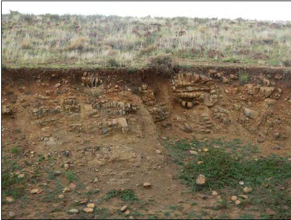
Figure 32. Quarry exposure of well-jointed, weathered dolerite bedrocks overlain by corestones and orange-brown lateritic soils, possible replacement site for Q1B near Winburg.
