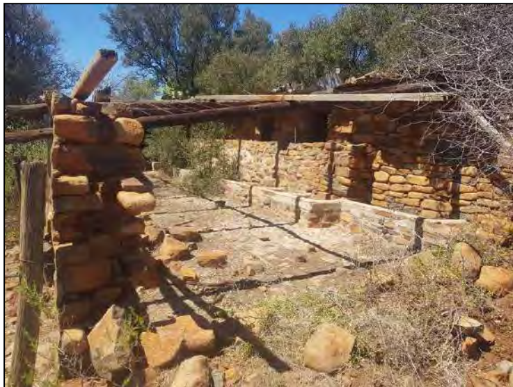
Figure 5-3: View of stone structure remains of livestock enclosures at Exigo-BP52.8-CP01.
