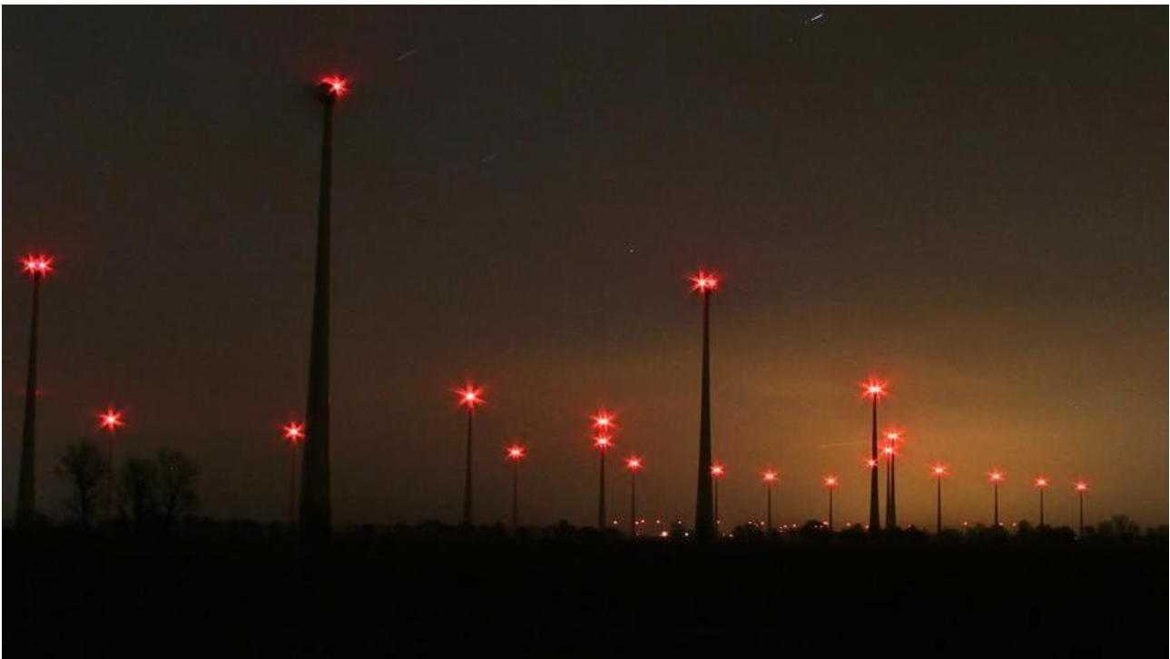
Figure 9: Example of aircraft warning lights fitted to the turbines as prescribed by the CAA 7
