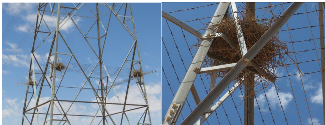
Figure 10: Pied Crow nest on Anti-climb fences.
