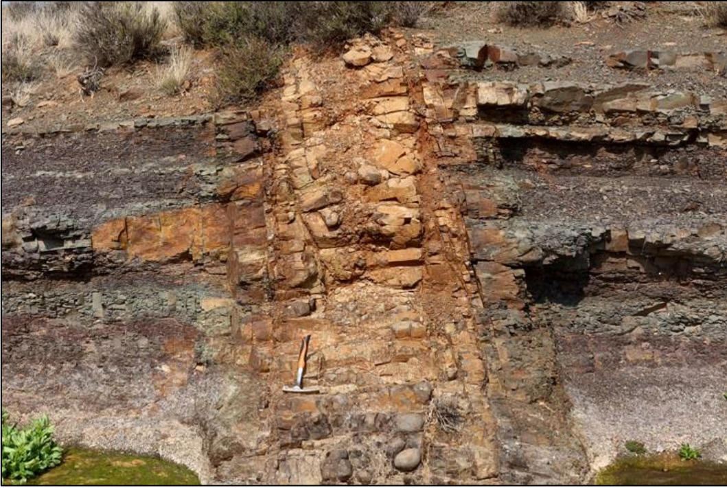
Figure 40: Narrow subvertical dyke of Karoo dolerite intruding Poortjie Member mudrocks showing clear cooled and baked margins, riverbank section near Spes Bona farmstead on Farm 3/200 (hammer = 30 cm).
