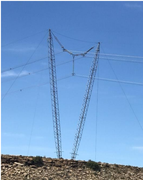
Figure 12: Pylon design that provide fewer opportunities for nesting sites.
