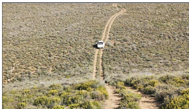
Figure 72: Typical two-track type farm road.
