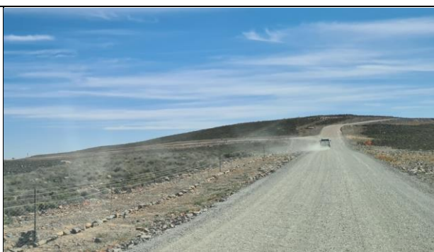
Figure 73: Typical WEF constructed access road.
