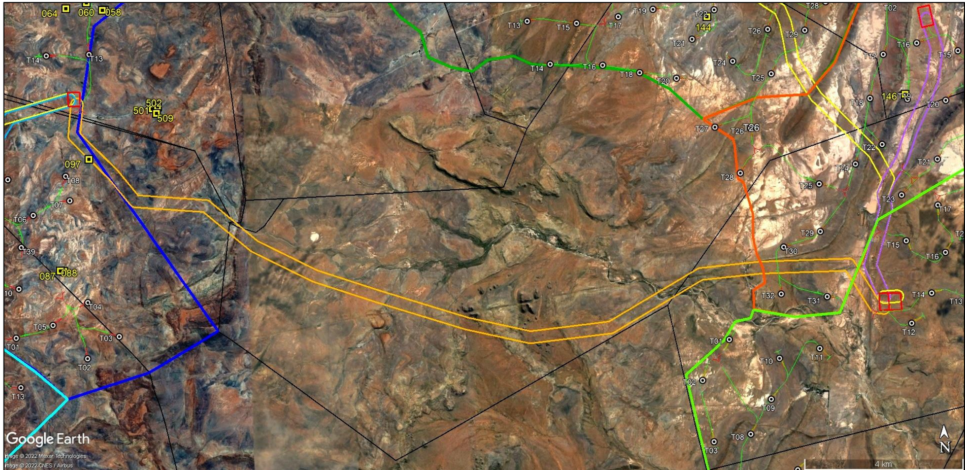
Figure A1.7: GoogleEarth© satellite image showing the 300m wide 400 kV powerline corridor (orange) connecting the Taibos collector substation in the west and the Soutrivier collector substation in the east (red rectangles). Fossil site Loc. 097 refers to scrappy plant remains of low scientific and conservation value for which no mitigation is recommended. Very little time was spent within the 400 kV powerline corridor during the reconnaissance-level site visits so a pre-construction palaeontological walkdown of the authorised powerline footprint here is essential.
