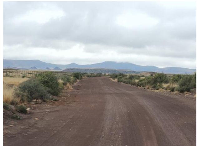
Figure 56: Typical transformation associated with an unpaved gravel road.
