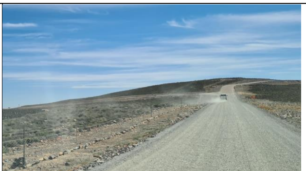
Figure 73: Typical WEF constructed access road.
