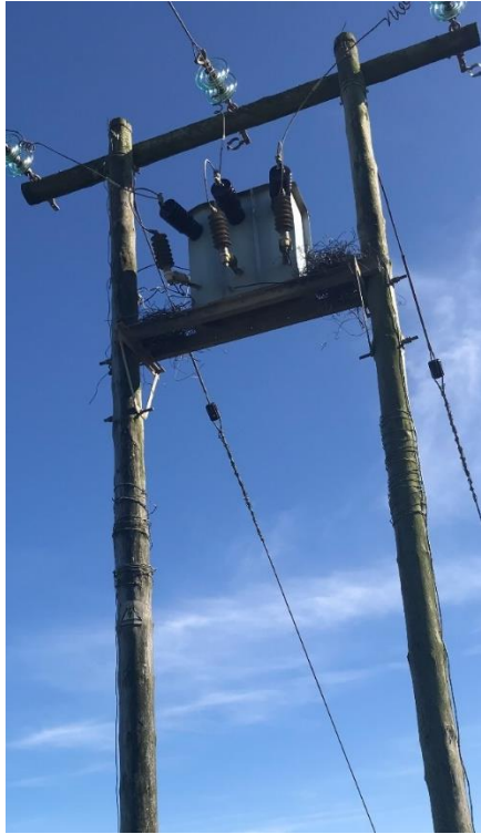
Figure 11: Crow nests constructed entirely out of wire may become a fire hazard.
