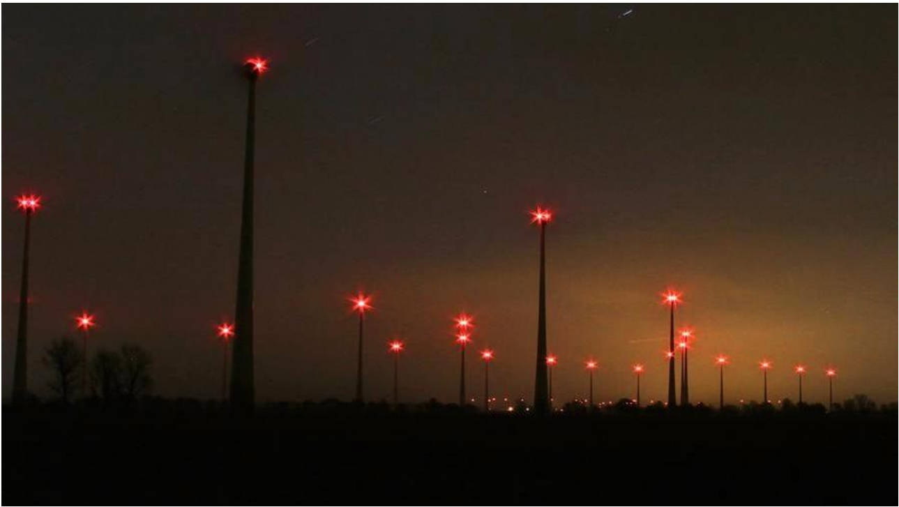
Figure 9: Example of aircraft warning lights fitted to the turbines as prescribed by the CAA 6
