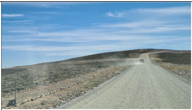
Figure 73: Typical WEF constructed access road.
