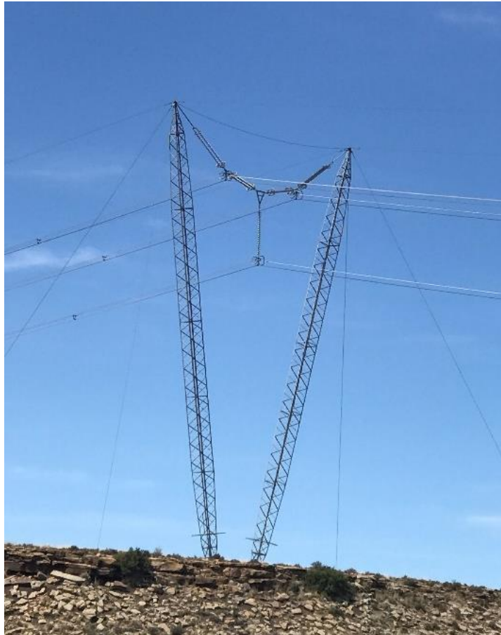
Figure 7: Pylon design that provide fewer opportunities for nesting sites.
