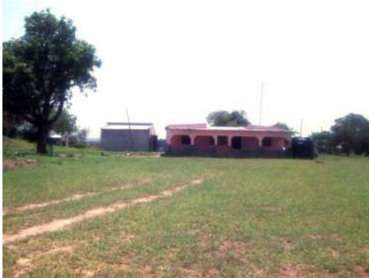
Plate 5.3 – A typical permanent house constructed of concrete (site 1171)
