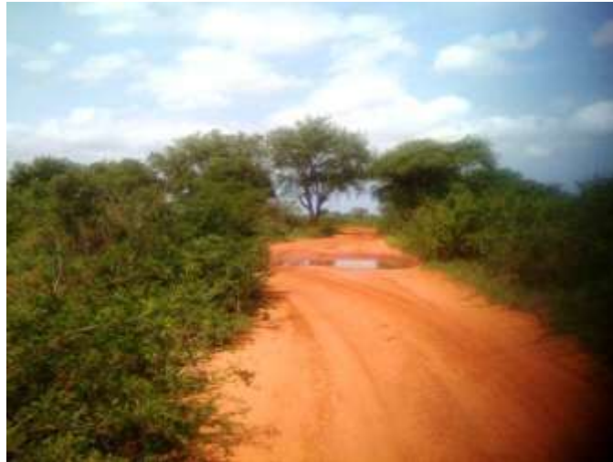
Plate 5.2 - The road from Catembe and Boane is in a very poor state
