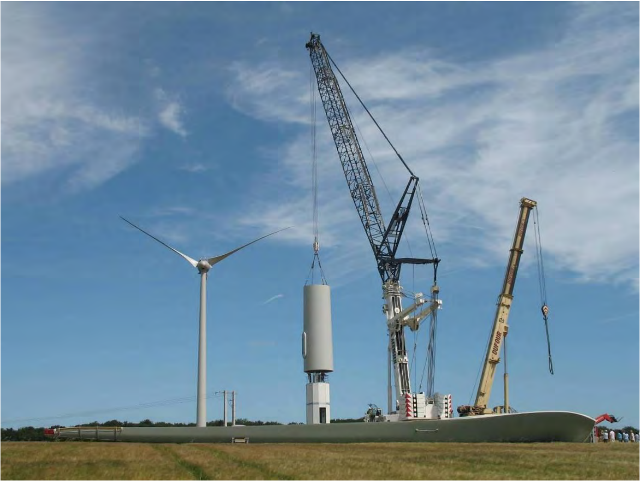
Plate 2.1: Assembly and erection of the tower sections
