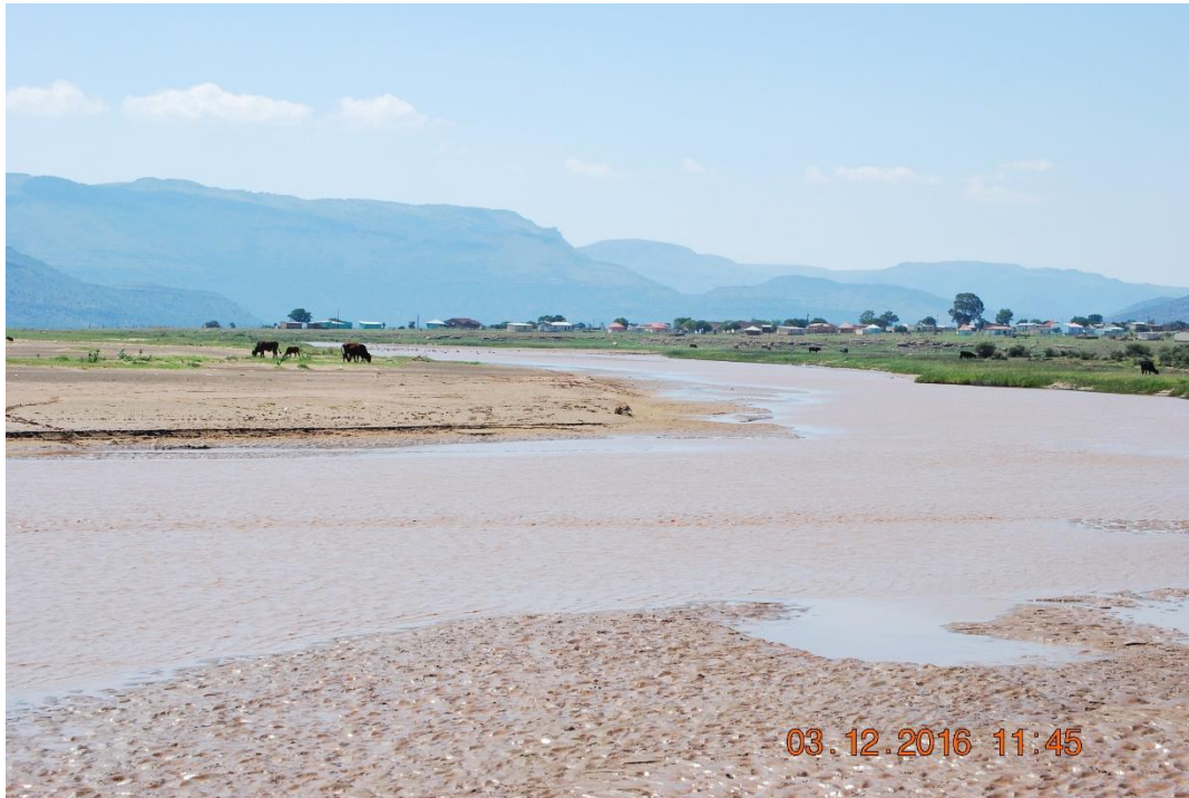
Plate 1: A view of the proposed mining area, showing the accumulation of sediment within the main channel and banks
